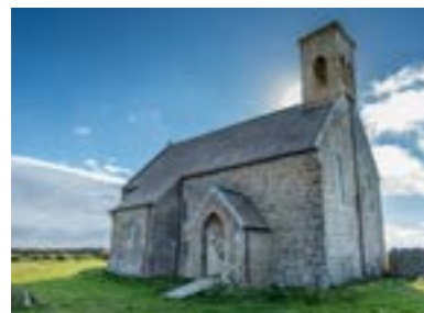
Flimston Chapel Pembroke, SA71 6EB
