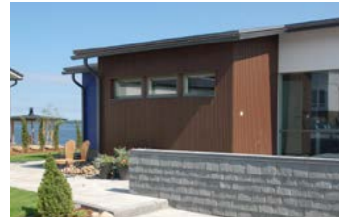
Private residence, Helsinki, Finland
