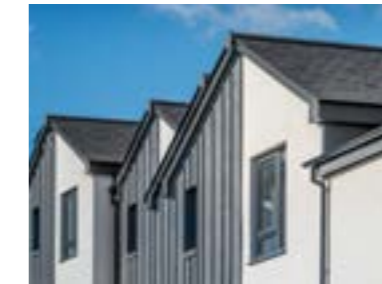
The Courtyard Pavilion Rise, St Austell, PL26 6DH
